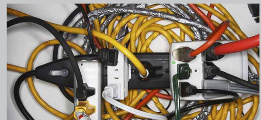
overused powerstrips & improper use of extension cords
