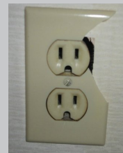
damaged/missing outlet faceplates
