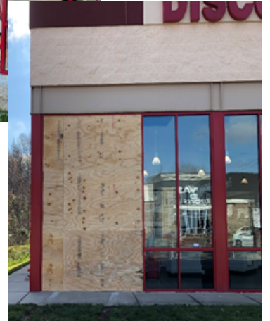
Example of outside damage and boarding up
